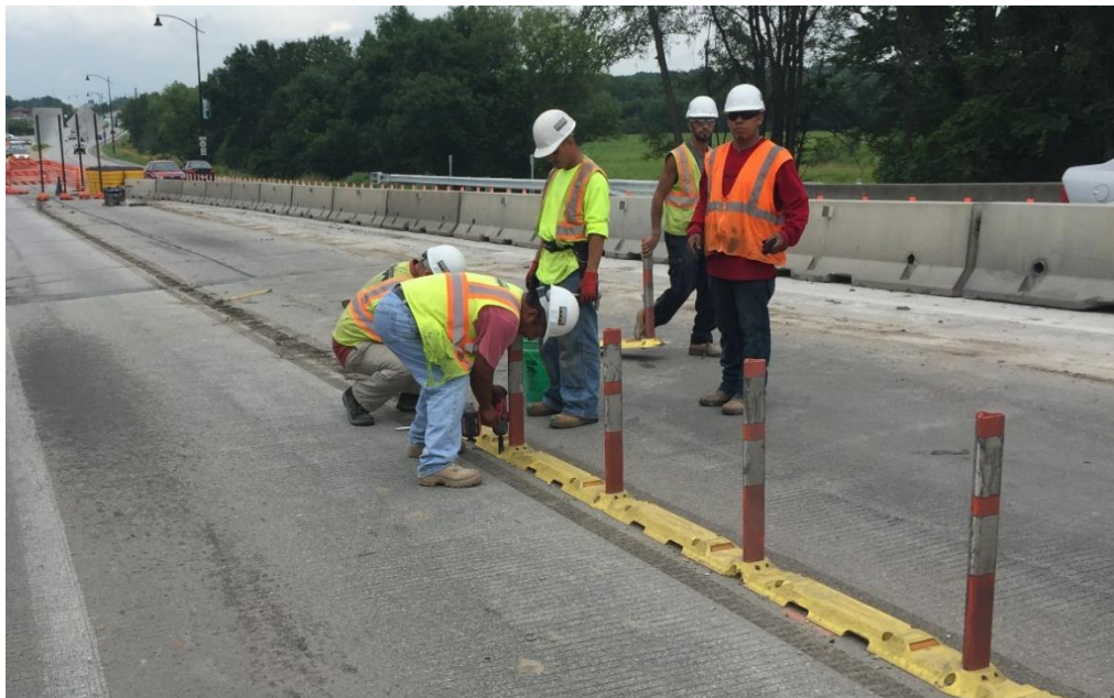
Figure 1. Temporary bollards being detached by workers
