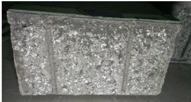
c) Bond interface (overlay concrete)
