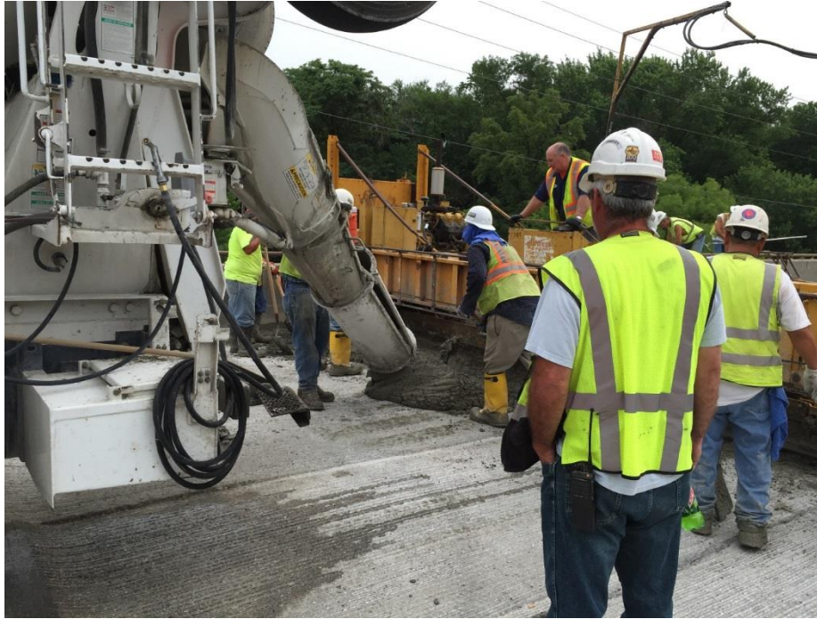
Figure 6. Ready-mixed concrete being placed on the deck
