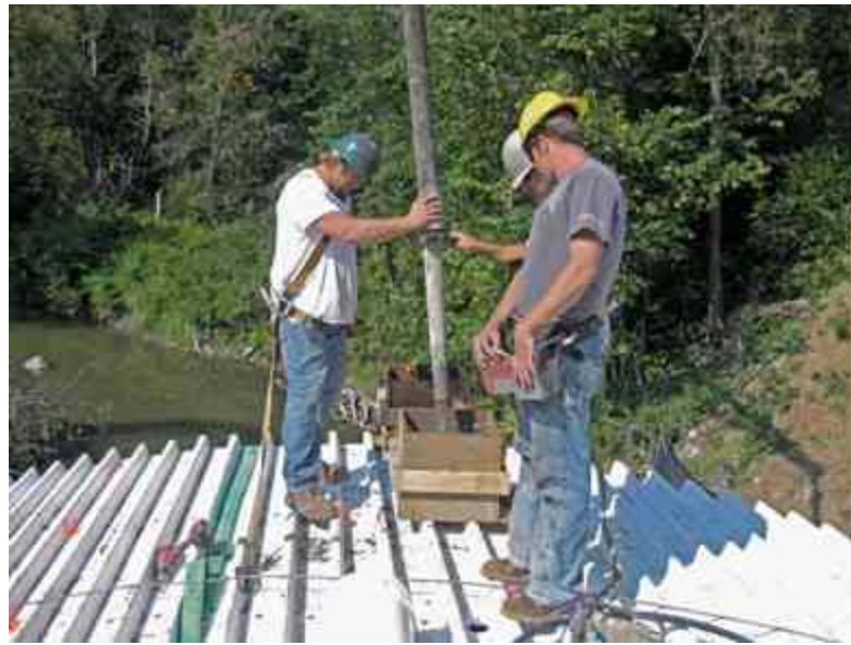
Workers are pouring concrete into FRP tube arches for the Royal River Bridge, constructed in Auburn, ME.
