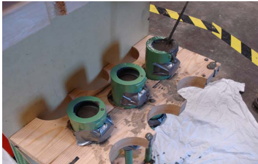
Figure 3.5 Rodding grout in #6 NMB splices
