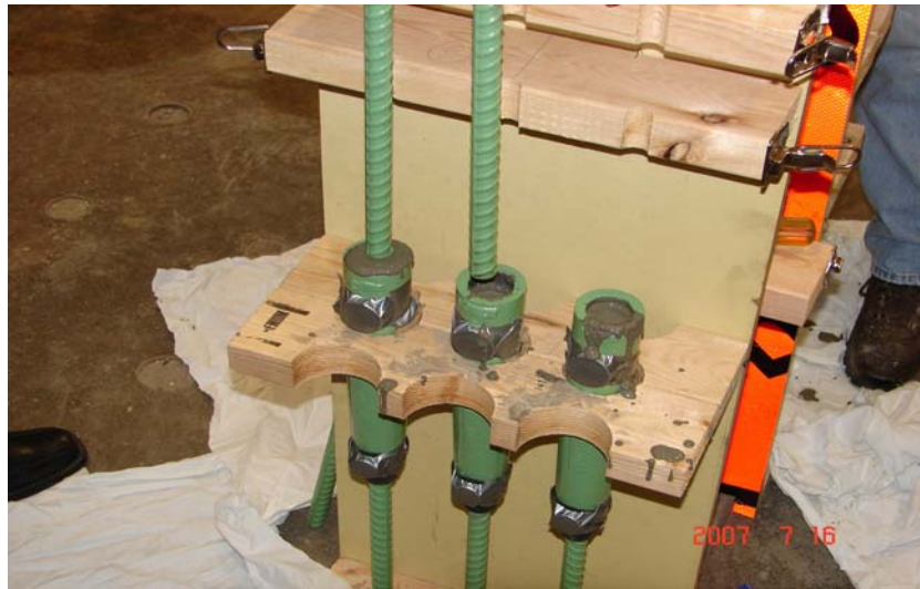
Figure 3.6 Inserting #6 bars in NMB splices
