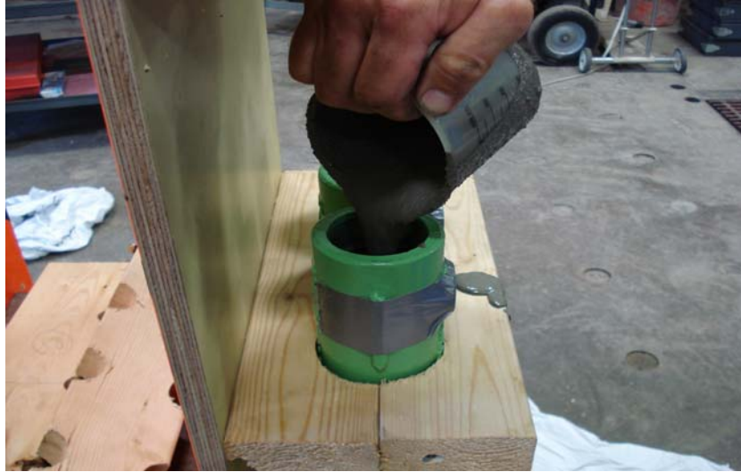
Figure 3.4 Pouring grout in #11 NMB splices
