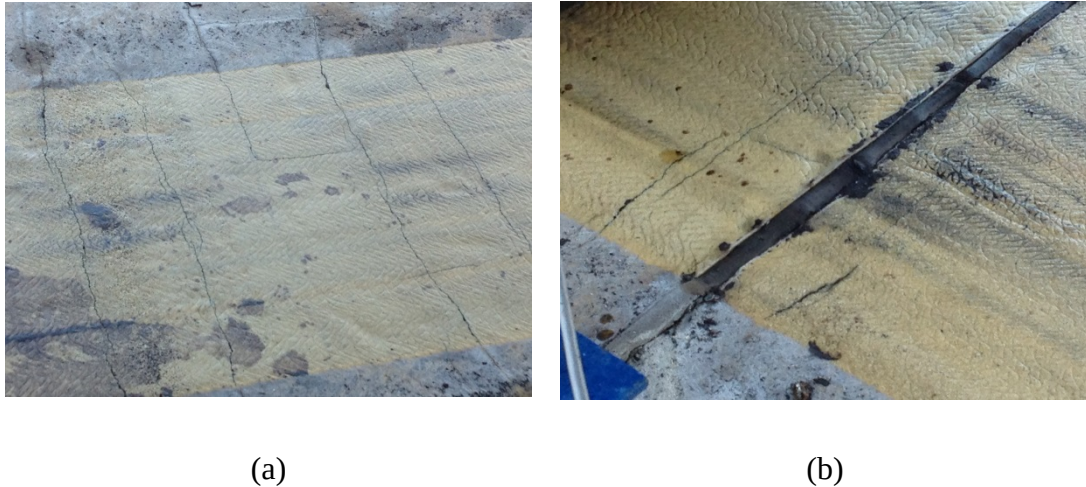
Figure 5.7 Cracks on (a) at Mid-Span, and (b) at the connection
